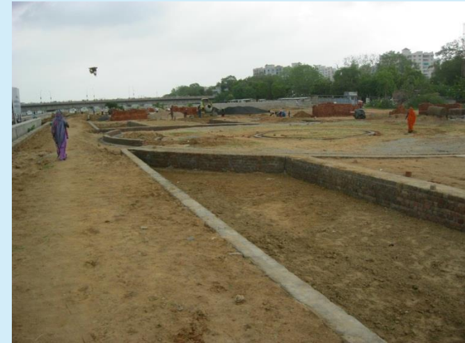
Native soil at the bottom of storm water planter
