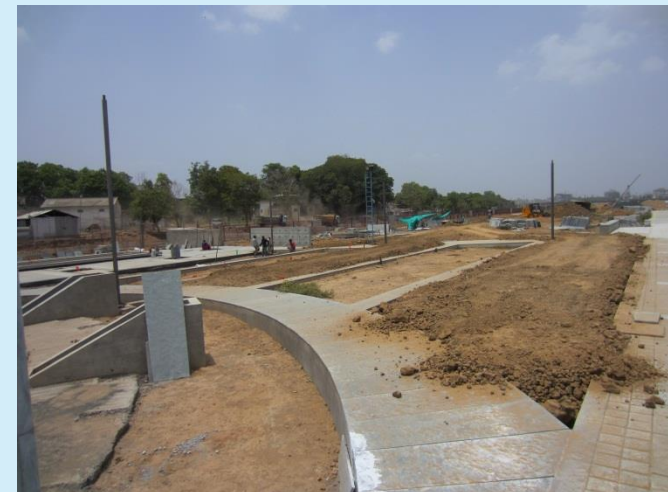
The storm water planter filled with aggregates, sand and top soil.
